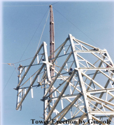
Tower Erection by Ginpole
