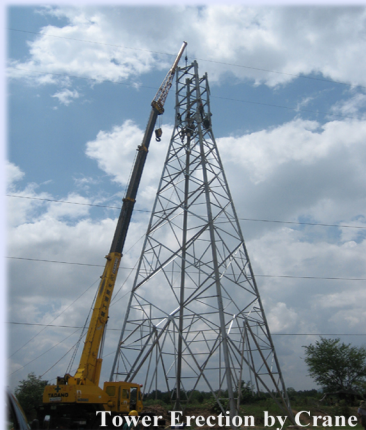
Tower Erection by Crane
