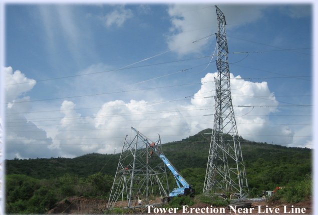
Tower Erection Near Live Line
